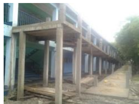
November: Construction of Ramp
